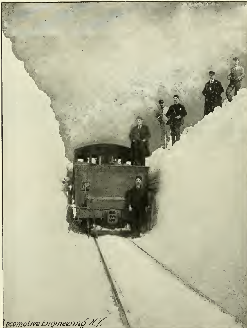
HANCOCK & CALUMET R.R., APRIL 1, 1893—NEAR ALLOUEZ STATION. SNOW OVER THE TELEGRAPH POLES, TUNNELED TO REPAIR THE WIRES.
